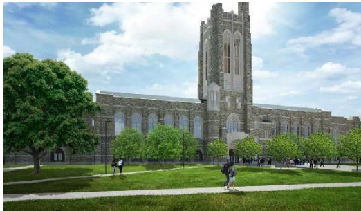
Existing City College Building
